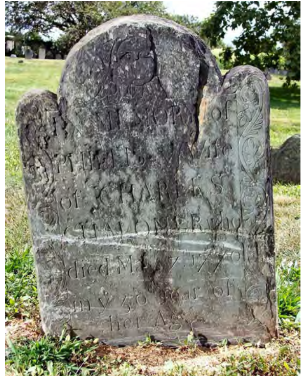
An example of the visually incompatible patching mortar (Marker 72). Looking at images soon after patching (see ) it appears as if the mortar never matched the stone well. The fill of the delamination crack at the lower portion of the image represents a good technique for repairing that condition but it should have also been employed in the delamination voids at the edges of the grave marker that instead consist of large areas of fills which are visually jarring and detract from the grave marker and inscription. Right: Marker 72 in 2008.
