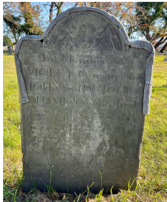
Marker 9 is currently the only gravestone that has a lead cap on it. This cap is breached in two locations so it is recommended to remove and perhaps re-cap depending on the condition of the slate underneath it. This is a viable repair option when caps are fitted and customized to each marker.
