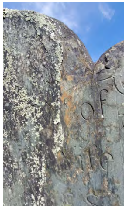
Left: marker 72 in 2020 prior to restoration. Right: a detail of the condition at the top right of the marker confirming the needlessly large unsightly patch that was implemented.
