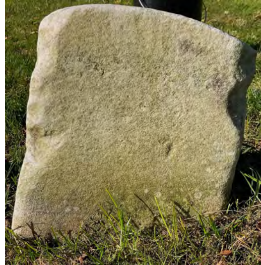
This marble marker exhibits several losses on its edges. Because it is low to the ground it is likely landscaping equipment has repeatedly impacted the marker. The appearance of the loss suggests it is older as it is weathered and soft at the edges.
