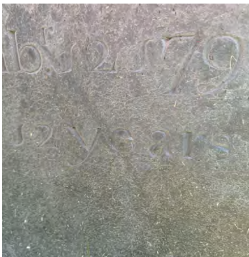
Example of flaked surface where flaking is densely stacked and not treatable. This is designated Severity I because it is on the majority of the front surface.
