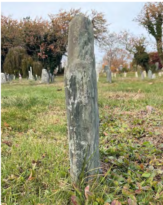
Example of Priority 4 Delamination – there are no treatable areas but the condition is extant.
