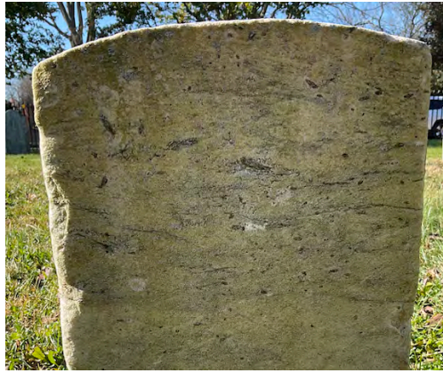
Marker 149 is an example of a marble with mild Disaggregation of a Severity of 4.
