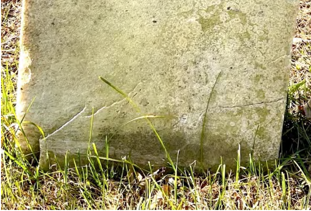
Marker 70 cracks in marble that require repair before additional loss of material results
