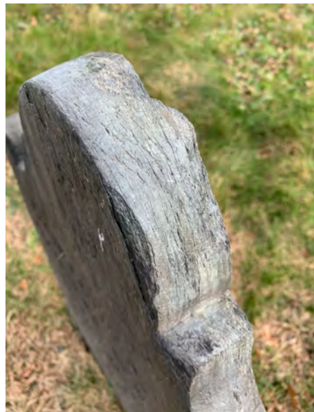
Examples of Priority I Delamination. The bottom right image depicts a grave marker that does not have a number of voids to fill and largely the top delamination is densely packed however there is a small area of delamination on the front that threatens the inscription and is wide enough to receive a fill. This could also be a candidate for a cap due to the intact nature of the top of the grave marker.
