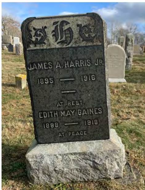
Marker 269 is a granite with Soiling of a Severity of 1.
