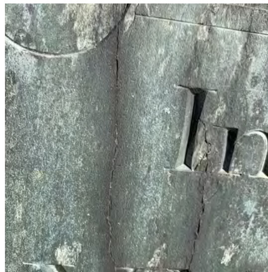
Marker with cracks that are too thin to fill. The dark discoloration on either side of the cracks is not moisture as in the image on the left but soiling that is attracted to the moisture the cracks hold.
