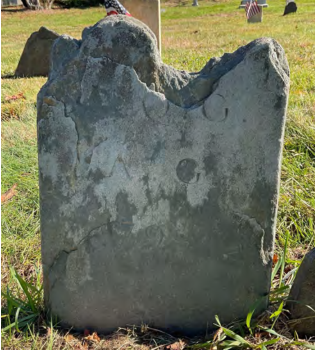
Example of Priority 2 Delamination that consist of treatable voids and gaps due to delamination/ The little legible inscription that remains is under threat of loss.
