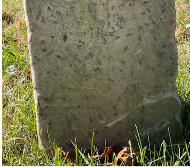
Marker 150 has multiple losses and fresh scrapes due to mechanical abrasion presumably from lawn equipment.
