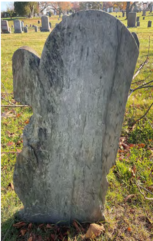
An example of loss typical of the majority of the slate grave markers: parts are missing in their entirety such as the very top of this marker and/or a significant layer of the slate is missing.
