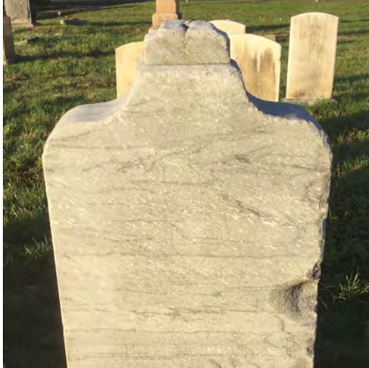
Examples of loss on marble grave markers: the top decorative element is missing (this is known because a pin is revealed) and there is loss on the right edge of the middle of the marker where it has been chipped.
