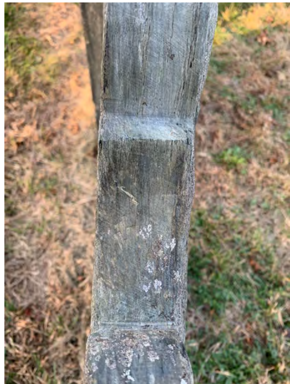
Evidence of another repair campaign on two different markers. This repair campaign does not have any associated documentation so the dates of execution are unknown. The delaminated tops of select markers have been tooled to relatively sound stone. It is an aggressive intervention but appears to have arrested the delamination.
