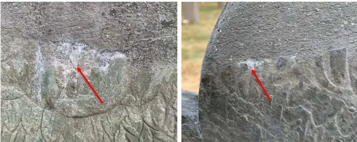
Markers 60 (left) and 81 (right) have efflorescence at the perimeter of a mortar repair.
