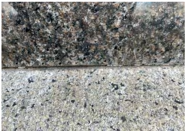
Example of an open joint in granite.
