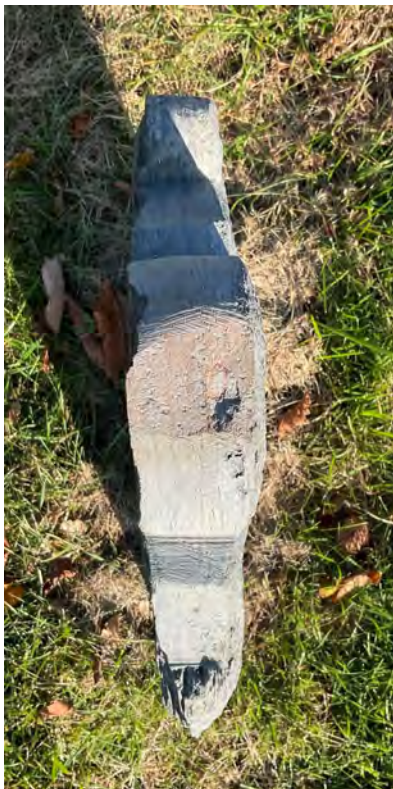
Evidence of another repair campaign on two different markers. This repair campaign does not have any associated documentation so the dates of execution are unknown. The delaminated tops of select markers have been tooled to relatively sound stone. It is an aggressive intervention but appears to have arrested the delamination.
