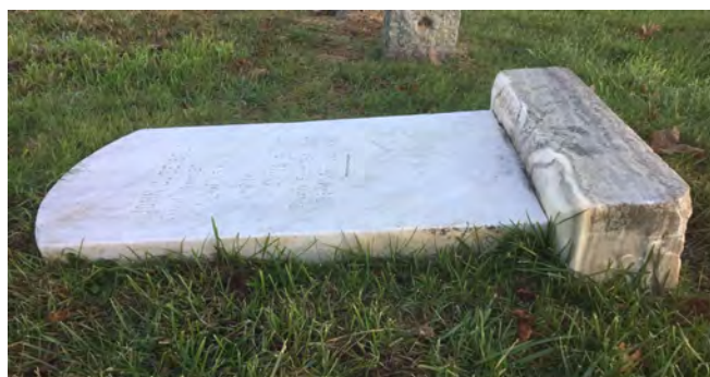
Marker 139 – the marker has fallen over due to unknown reasons. This would be a high priority to reset because there are new stresses and pressure points on the marker that may cause greater damage in the future.
