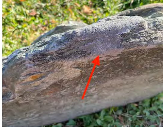
Marker 201 exhibits crustose lichens, a hard layer that looks like cement as a result of integration of minerals from the stone into the lichen structure.
