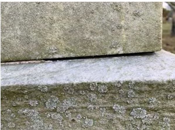
Example of an open joint in marble.
