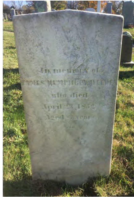
Markers 317 and 355 are typical examples of atmospheric soiling.
