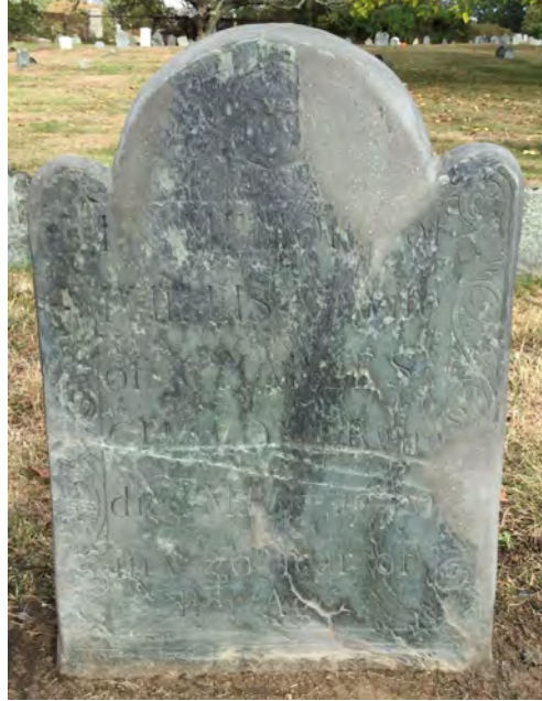
Marker 72 in 2020 shortly after its restoration: the patching mortar was visually jarring then as well. The color then somewhat matched the stone but the inclusions or aggregate of the patching mortar were already unsatisfactory.
