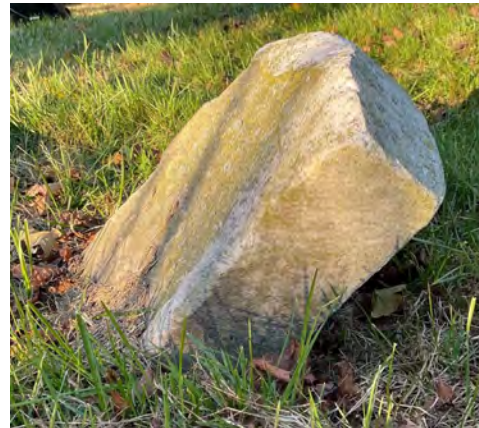
The marble though thicker warrants resetting due to its angle.
