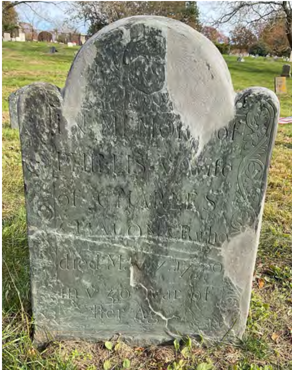
An example of the visually incompatible patching mortar (Marker 72). Looking at images soon after patching (see ) it appears as if the mortar never matched the stone well. The fill of the delamination crack at the lower portion of the image represents a good technique for repairing that condition but it should have also been employed in the delamination voids at the edges of the grave marker that instead consist of large areas of fills which are visually jarring and detract from the grave marker and inscription. Right: Marker 72 in 2008.
