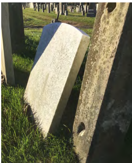
The marble marker being thin, at an acute angle to the ground and leaning towards a post warrants its resetting.
