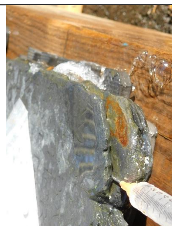
CBG MC-FC 12. DT. Flushing cracks with pressurized water.
