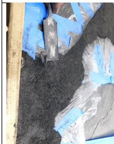
GLA 049 21. DT. Tooling Edison Coatings Systems 45 with Marine Latex in losses.
