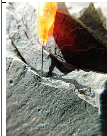
CBG MC-FC 17. DT. Injecting cracks with B-72.
