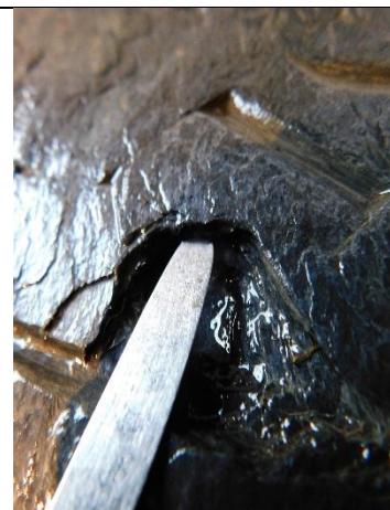
GLA 049 8. DT. Removal of roots from face carving.
