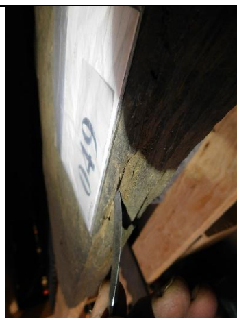
GLA 049 11. DT. Removing roots and earth between cleavage cracks before water contact.
