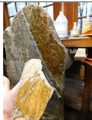
GLA 055 16. DT. Adhering proper left shoulder fragment with Akepox 2000.
