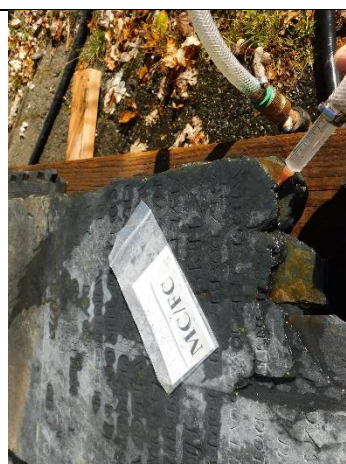
CBG MC-FC 11. DT. Flushing cracks with pressurized water.
