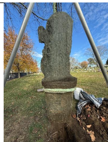
GLA 031 8. DT. Removal with tripod detail.
