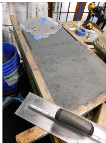
GLA 200 7. DT. Finishing cast section with Edison Coatings Systems 45 and Marine Latex.
