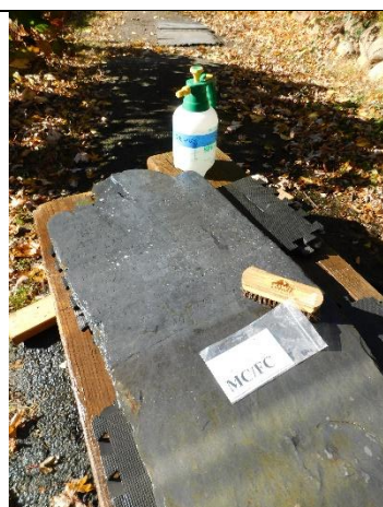
CBG MC-FC 10. DT. General cleaning with Orvus solution.
