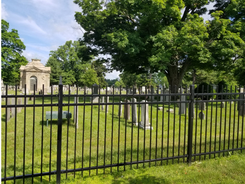
A steel picket fence installed around an historic cemetery. The spacing of the pickets allows passersby to view the cemetery. At the same time, the fence serves as a barrier.
